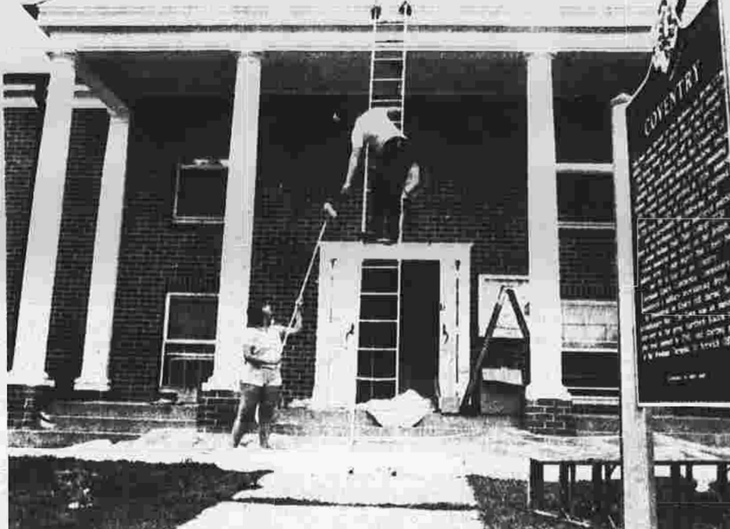
Town hall paint job
